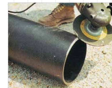
Fig. 5.11.4: Chamfering of DI pipe cut ends
